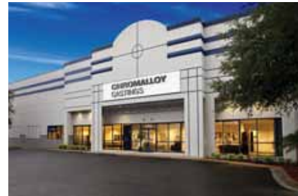
Courtesy of Chromalloy. Chromalloy Casting's new facility in Tampa, FL.
